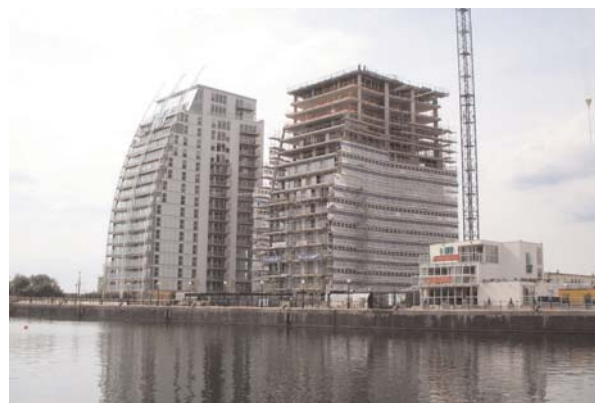
Exclusive apartments under construction in Salford Quays
