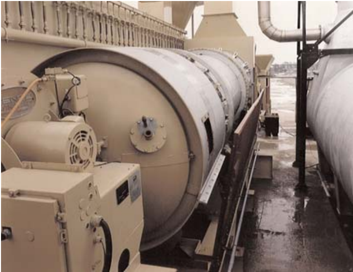
Close up of the thermal soil remediation unit.
