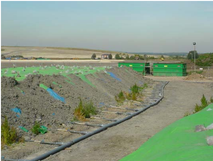
Side of the biopile showing aeration pipes
