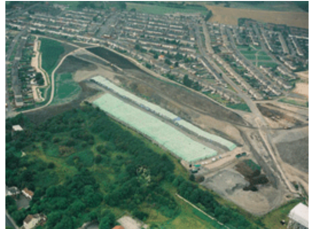
Aerial view of the two biopiles at Askern
