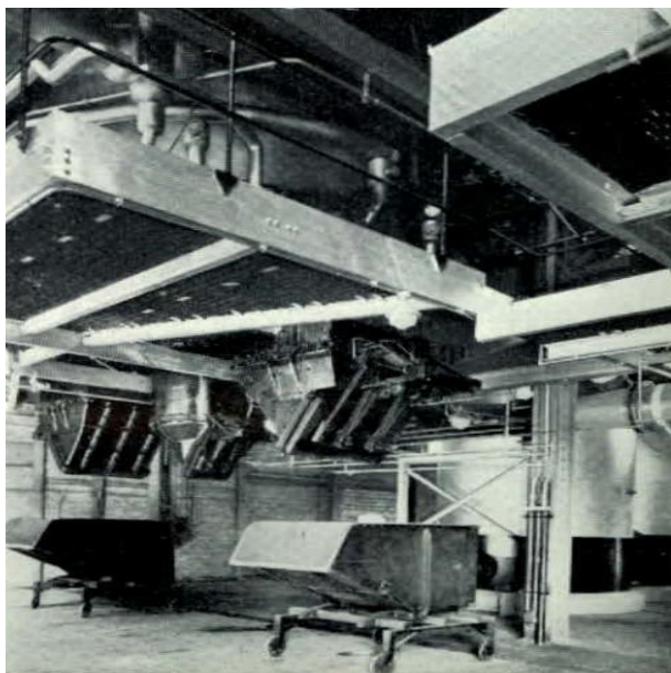
Photograph 14. The base of the H&G water gas plant installed at the former Southall Gasworks. Source: National Grid Gas Archive.
