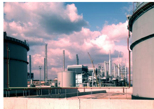
Photograph 13. Oil reforming plant at the former Tipton Gasworks. Source: National Grid Gas Archive.
