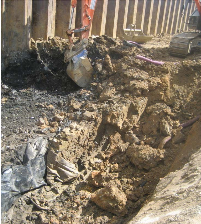
Separation and excavation of landfill material
