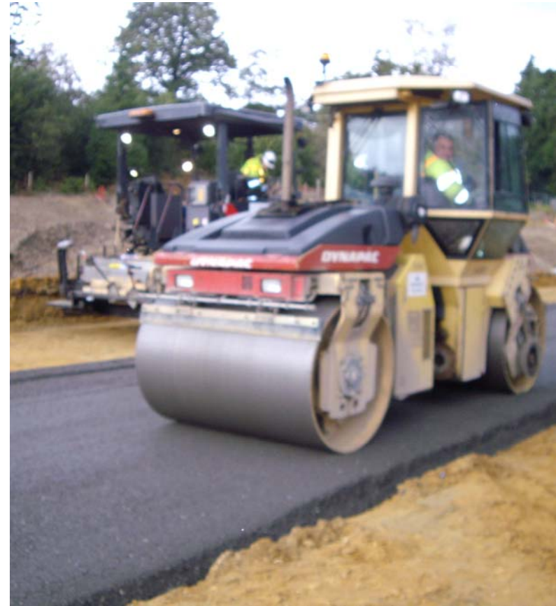
Compaction of foamix base
