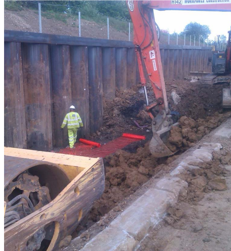
Indicator layer installed prior to backfilling with clean material for installing services
