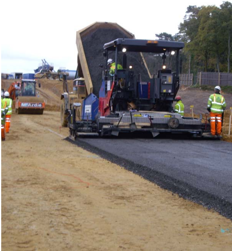
Laying of foamix base
