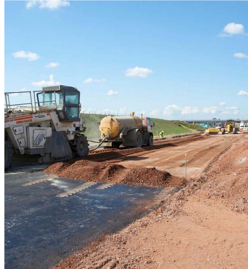
In-situ treatment of composite aggregate (planings and granite) to form bound road foundation
